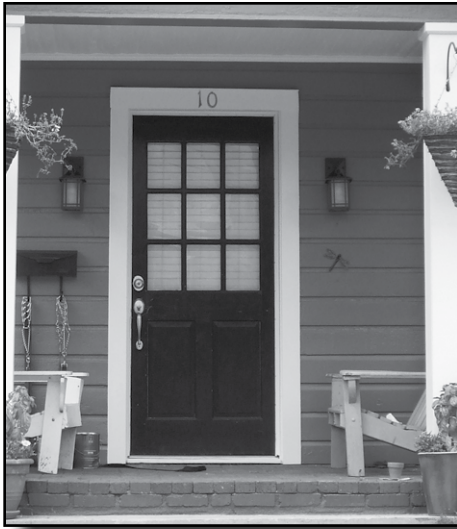
Doors are major character defining features.
