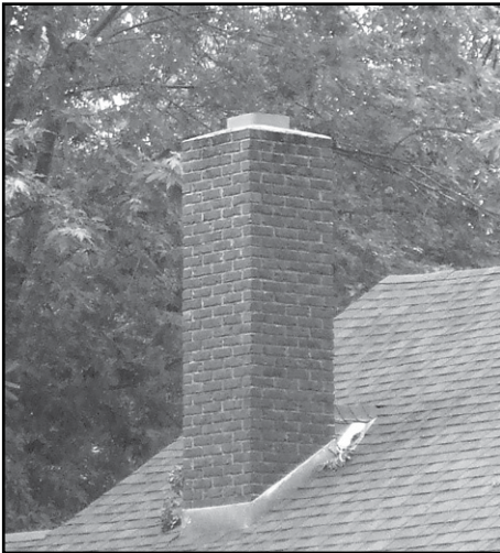
Typical Terra Cotta Chimney Cap
