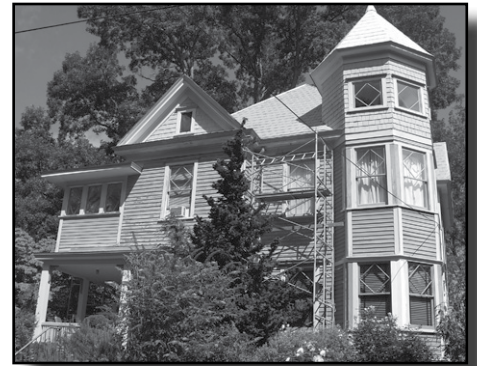
Example of a Minor Work project underway
