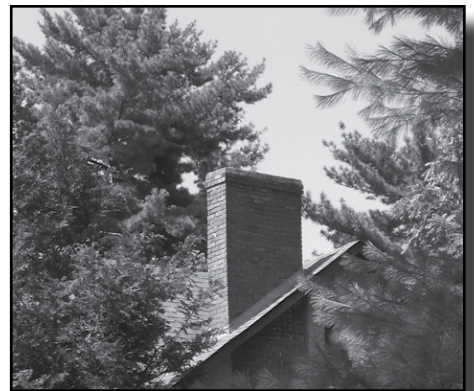
Concrete Chimney Cap
