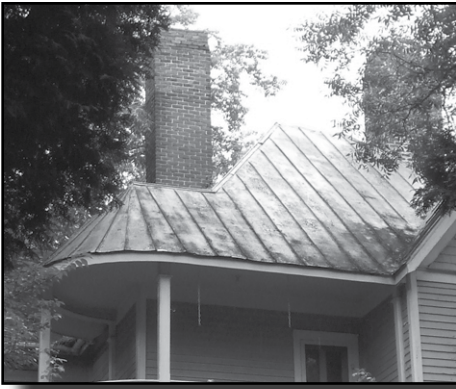
Standing Seam Metal Roof
