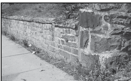
Stone Retaining Wall
