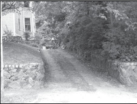
Pervious Driveways Reduce Runoff
