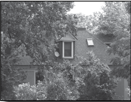
Locate skylights and satellite dishes in inconspicuous locations on a rear facing roof.
