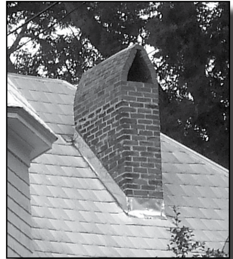
Brick Chimney Cap
